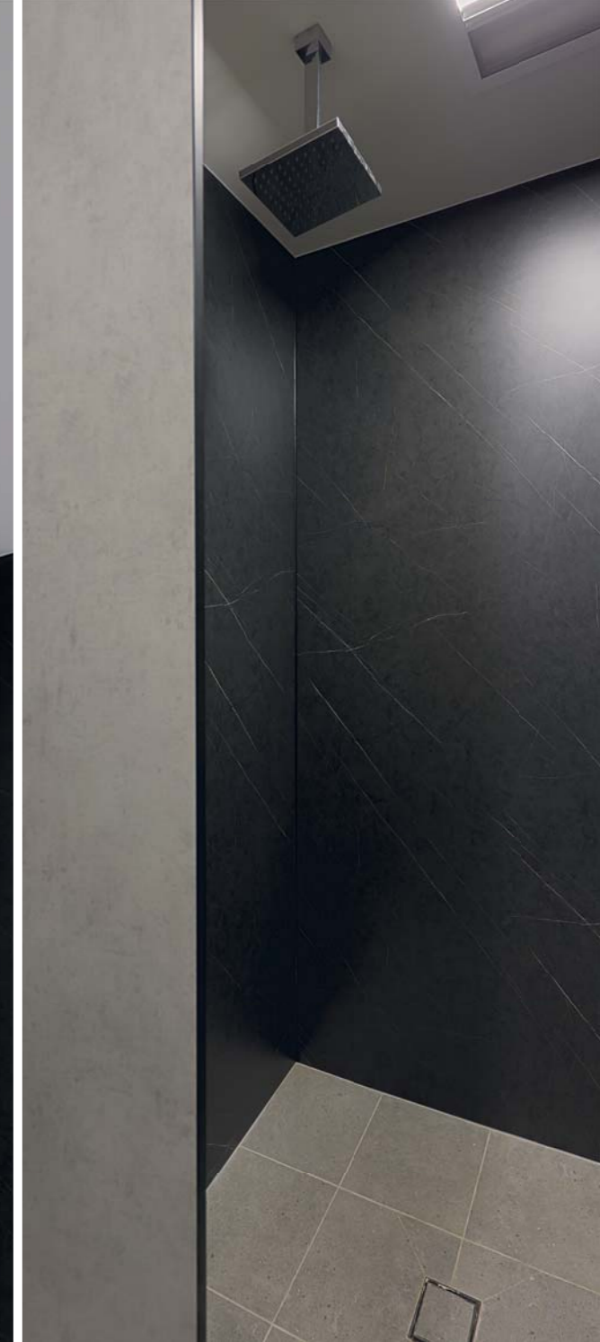
Wall panels in 5mm COMPACT laminate Athena Stone Smooth. Partition and seating in 13mm COMPACT laminate Grey Cement Smooth.
