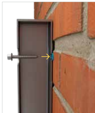
2 Drill rear wall of post with required diameter for fixing and then fix post to wall. Insert appropriate fixing into the wall for affixing post
