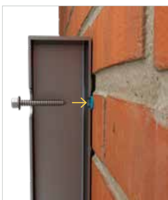
2 Drill rear wall of post with required diameter for fixing and then fix post to wall. Insert appropriate fixing into the wall for affixing post
