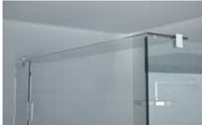
Provides rigidity for hinge panel supporting the shower door and return panel
